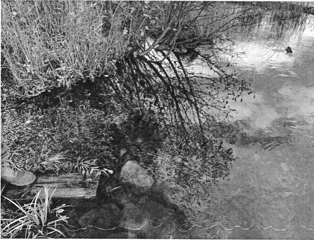
PHOTOGRAPH 5— View of right abutment area
