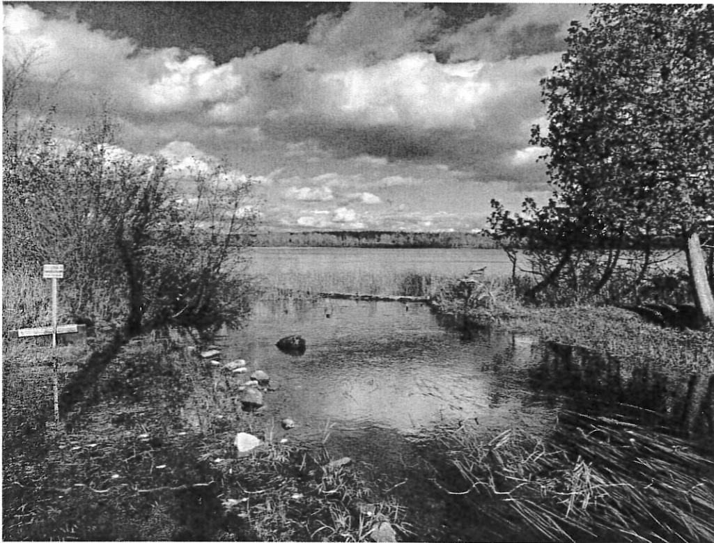
PHOTOGRAPH 1— Structure viewed from downstream
