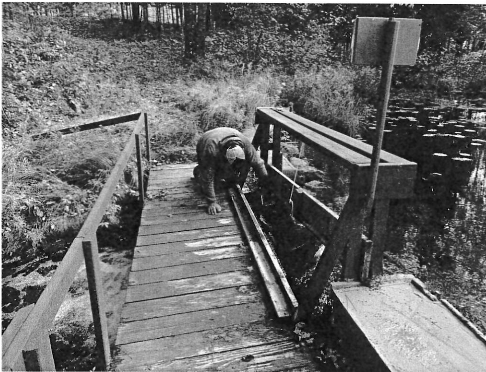
PHOTOGRAPH 4—Close view of spillway/stoplog section
