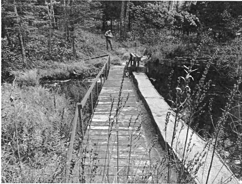
PHOTOGRAPH 7—Structure viewed from left abutment
