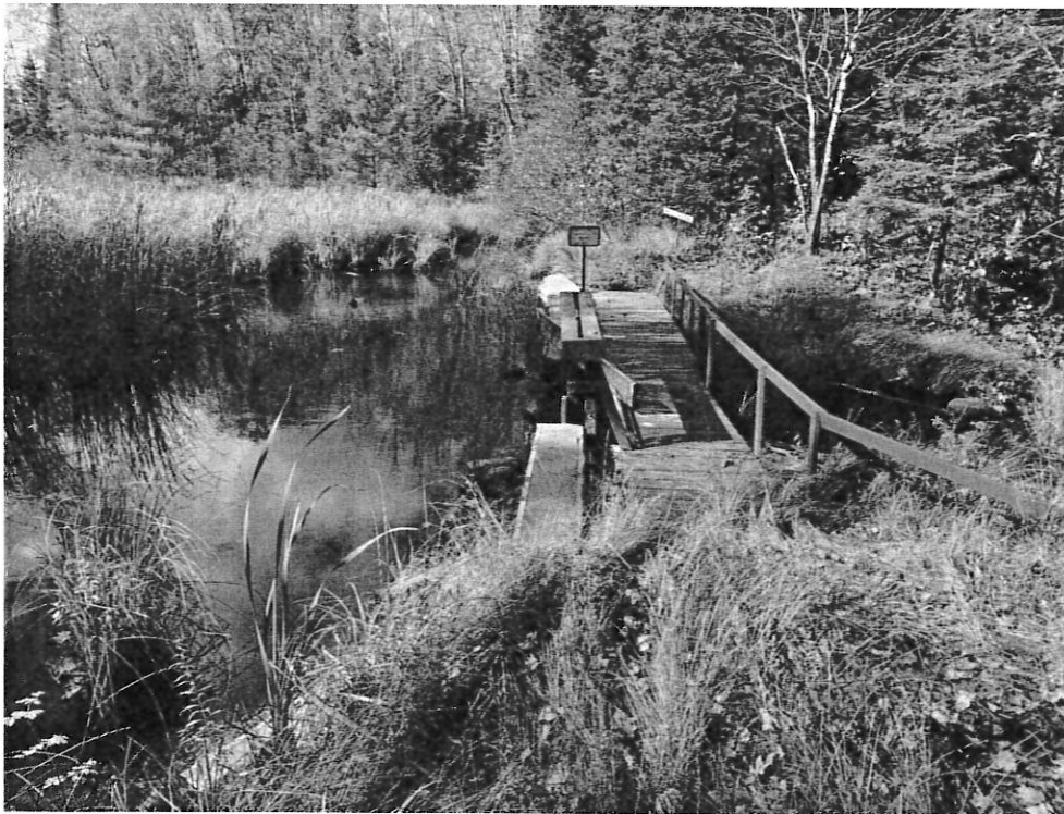
PHOTOGRAPH 2—View from right abutment
