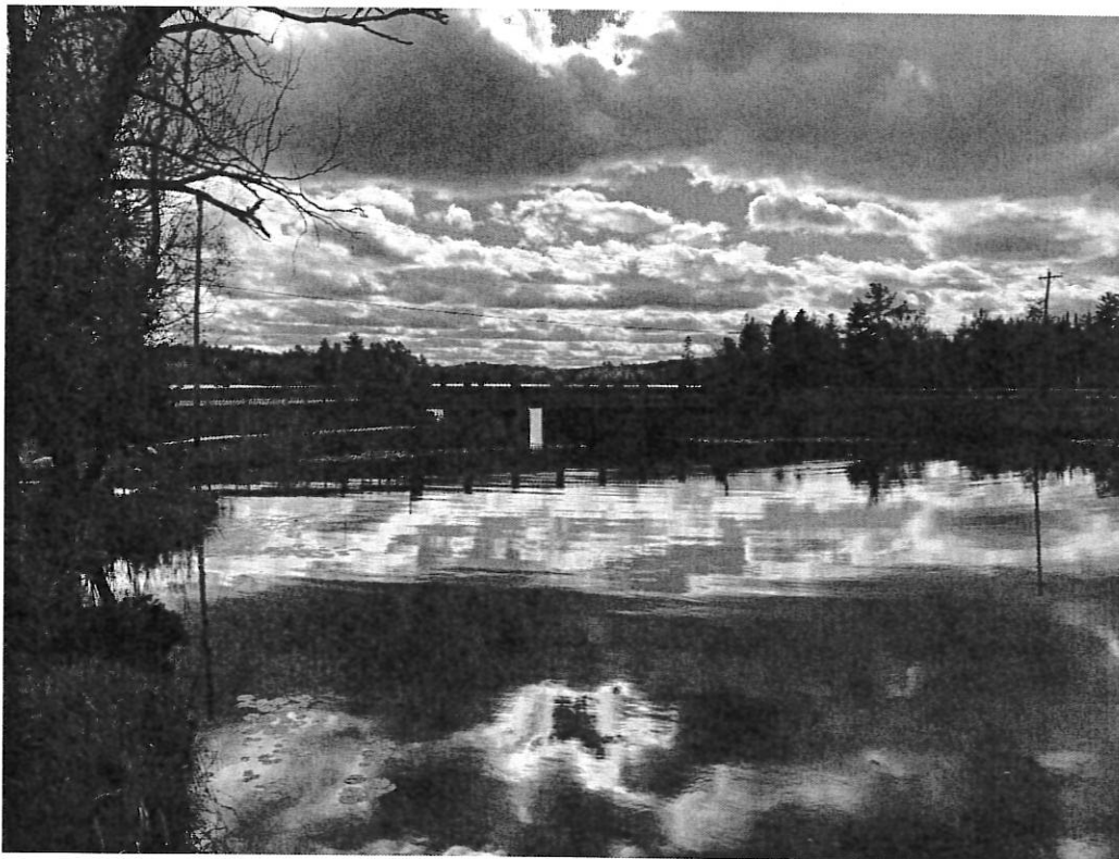
PHOTOGRAPH 8—US-2 bridge with elevation gage
