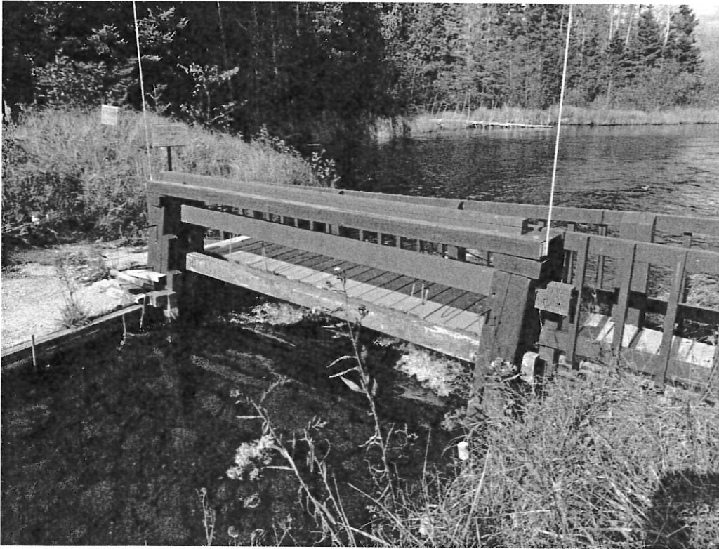
PHOTOGRAPH 5— View of spillway/stoplog section and inlet channel
