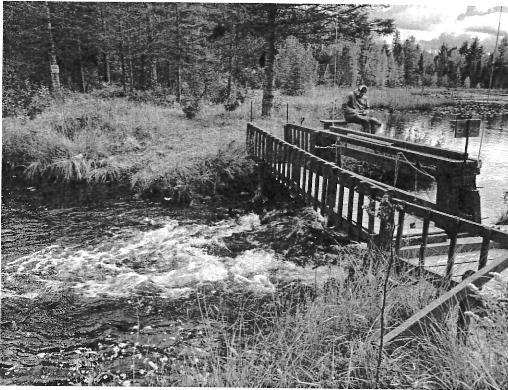
PHOTOGRAPH 7— View of downstream face and outlet channel
