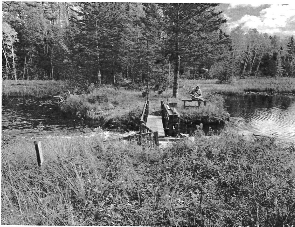
PHOTOGRAPH 2—View from left abutment
