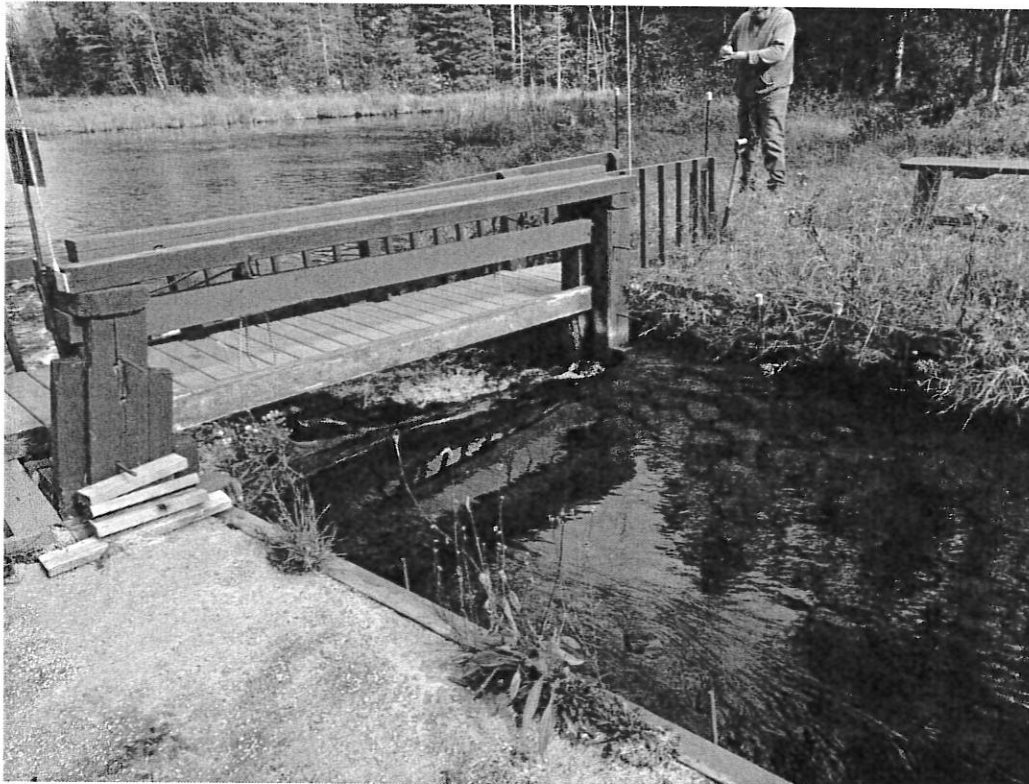
PHOTOGRAPH 4—View of spillway/stolog section and inlet channel
