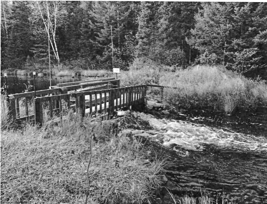
PHOTOGRAPH 6—View of downstream face and outlet channel
